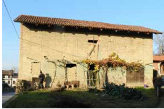
Figure 3 . Rural building in Priocca (Cuneo) with fired brick structure and adobe walls (credits Manuela Mattone)
